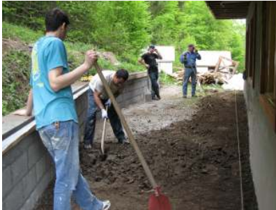
Preparing for new Patio Area
